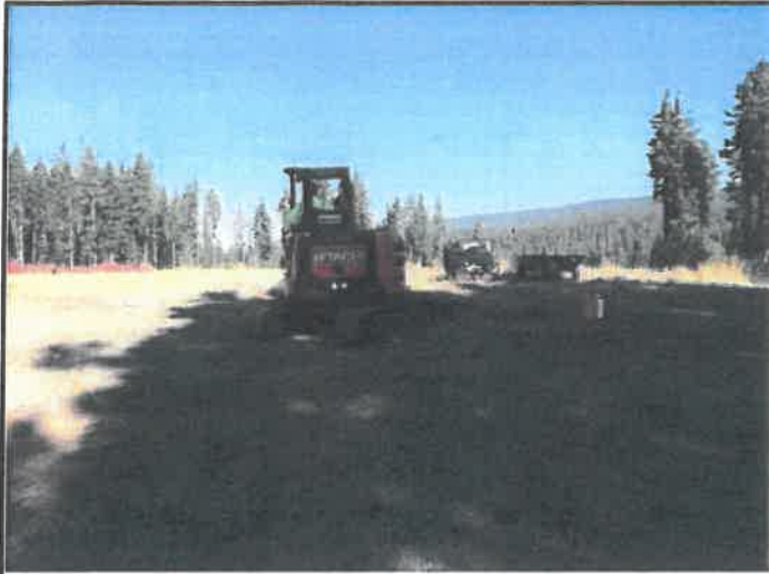
Excavation of test-pit TP-1 in Area 1 looking northeast
