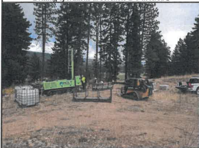
Drilling operations at borehole B-4 in Area 1
