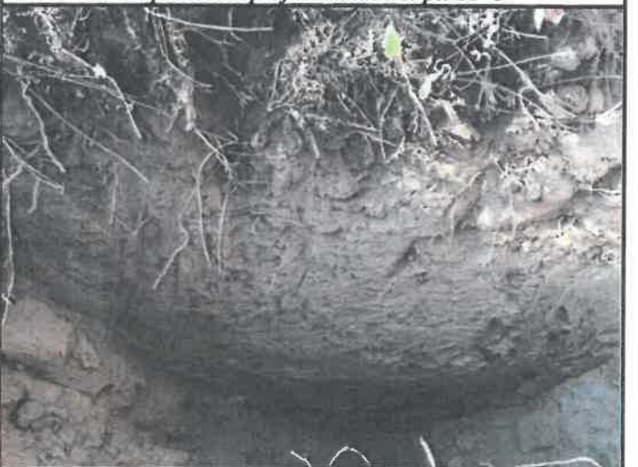
Exposed soil profile within test-pit TP-9
