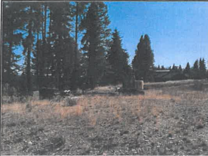
Excavation of test-pit TP-4 in Area 1 looking southeast
