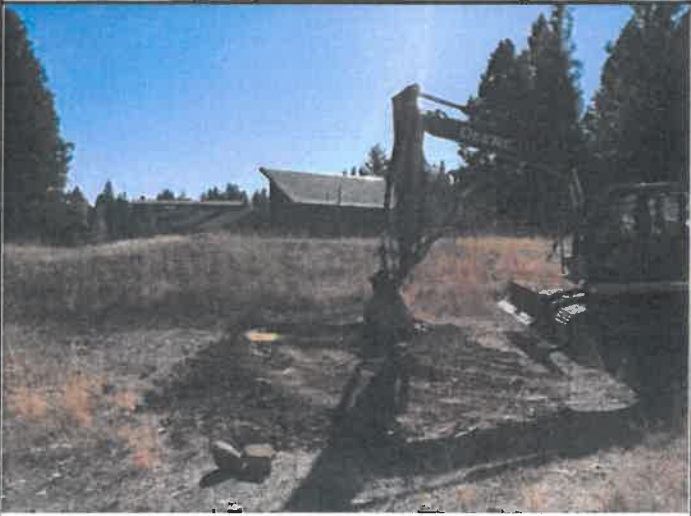
Excavation of test-pit TP-2 in Area 1 looking southeast
