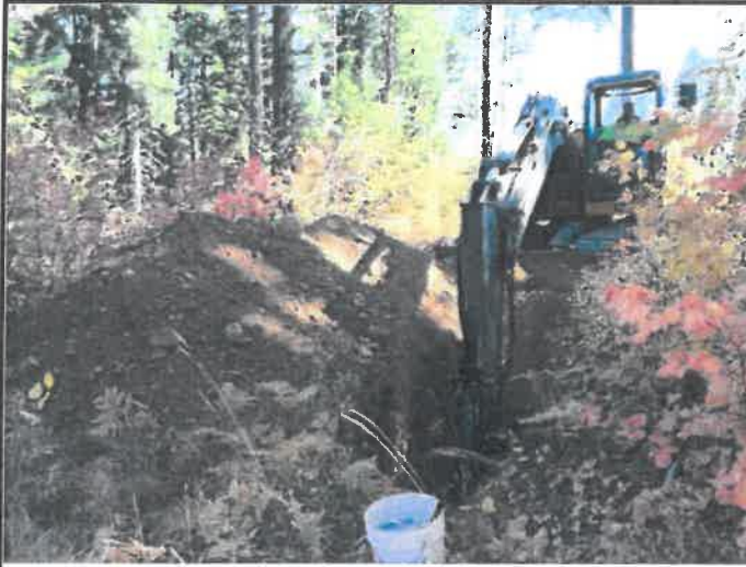
Excavation of test-pit TP-7 in Area 1
