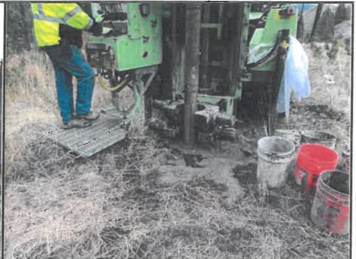
Drilling operations at borehole B-1 in Area 1
