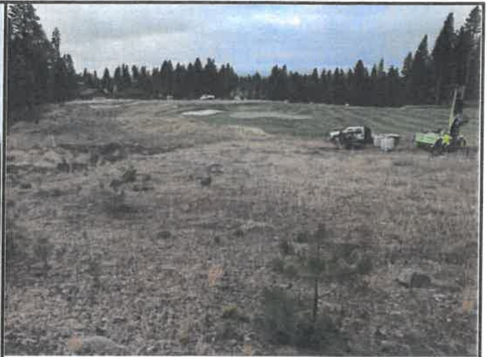
View of site conditions at Area 1 looking east
