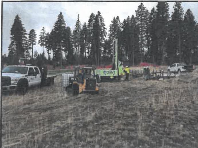
Drilling operations at borehole B-3 in Area 1
