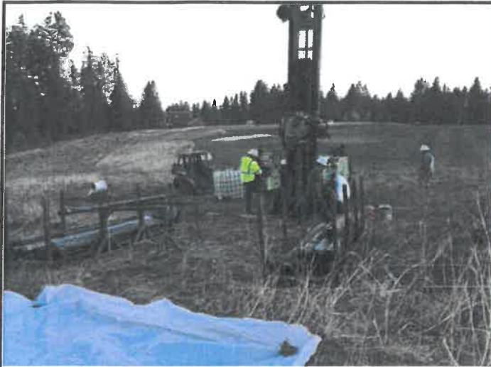
Drilling operations at borehole B-1 in Area 1
